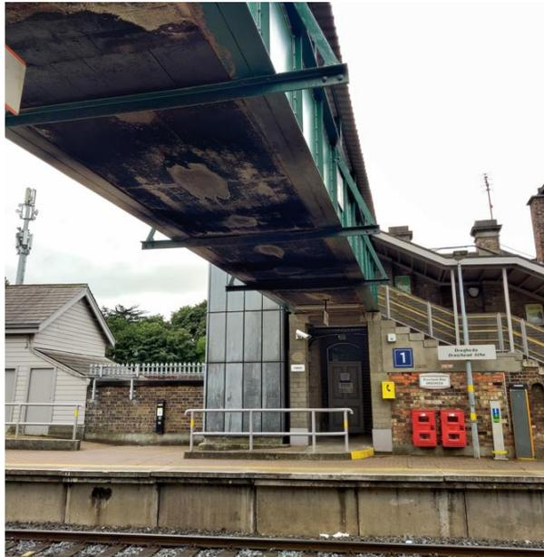
**Figure 6: Soffit of existing bridge showing steel sections beneath soffit**
